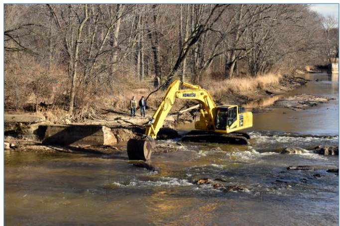
Demolition of the failed Collamer Dam in the Eel River, January
