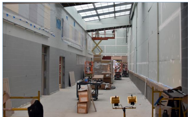
Construction in a hallway of the new high school, March
