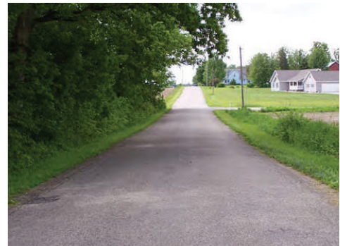
South County Road 300 West is an example of a local road.
