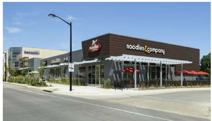
Top: Example built form existing in Whitley County. Middle and bottom: Example built form from other communities.
