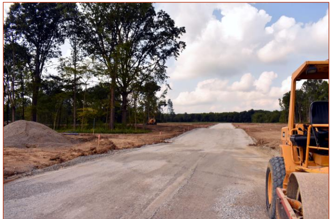
Development of streets in Ravenwood Section II, August, Columbia City.
