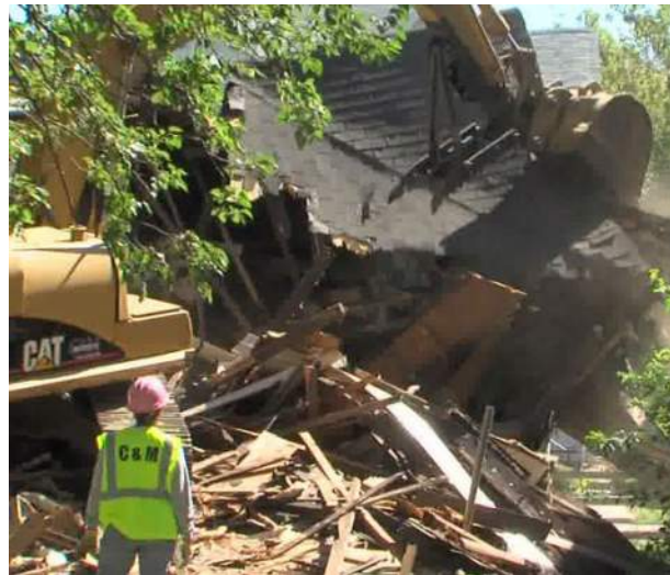
Figure 5i: Unsafe home being demolished
